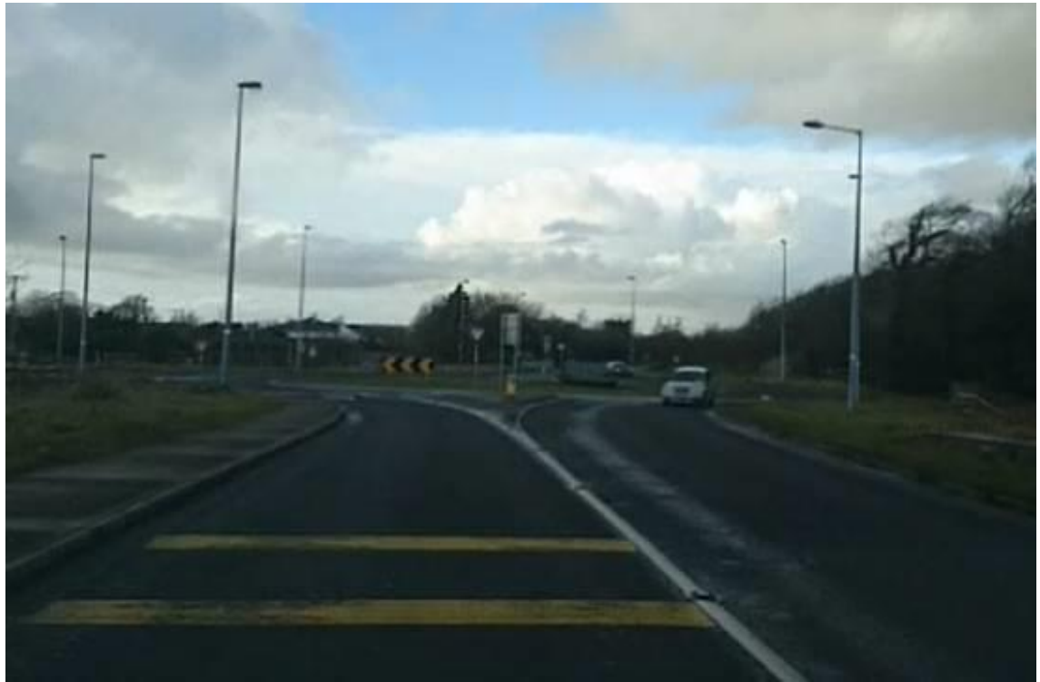
Figure 4: Northbound Approach to roundabout on N67
